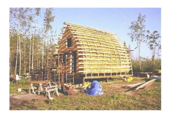
Figure 1: The vault cabin at Kissimmee Lake site, near Shell Lake, Saskatchewan
